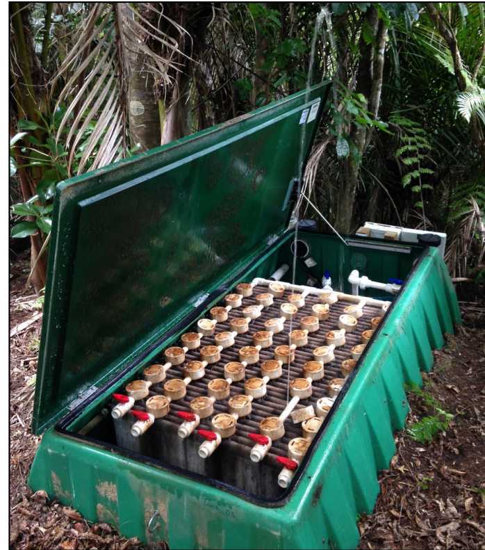
Orifices Check squirt height
